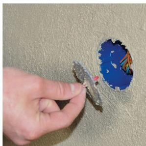
Remove the cleaning spring and mill
