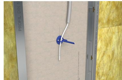
Fasten pipe support to drywall and guide lines or pipes through brackets through brackets.
