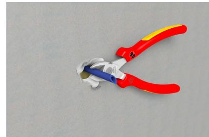
Use pliers to pinch the cable support to the wall.
